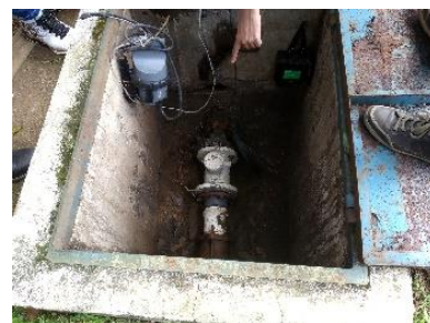
Figure 11. Water pipe installation to be measured by the prototype.
