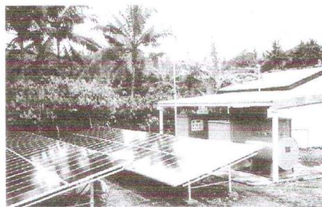
Gambar 3. Sistem *hybrid* PLTS dan diesel [1]
