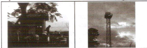
Figure 1: ISRA Radar Station in Merak.
